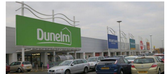
Park post refurbishment
